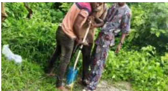
Technicians working on the borehole at Owena Core-trial site (Photo credit: CRIN - Owena)
