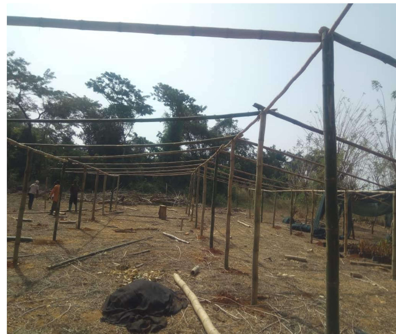
Construction of nursery shed.
