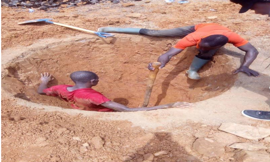
Figure 4 Constructing the “Kon-tiki” kiln at CRIG farms.
